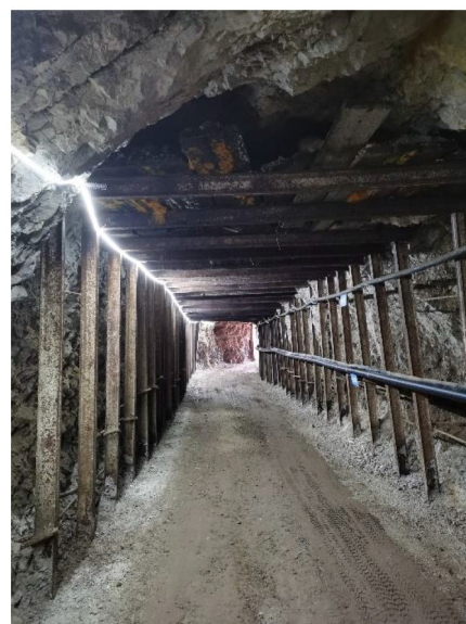
(b) 硐口段钢拱架支护
